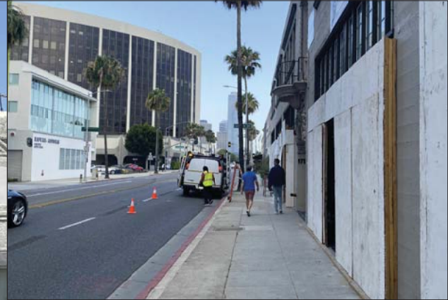
ADJACENT BLDG. 9701 UNDER REMODELING
