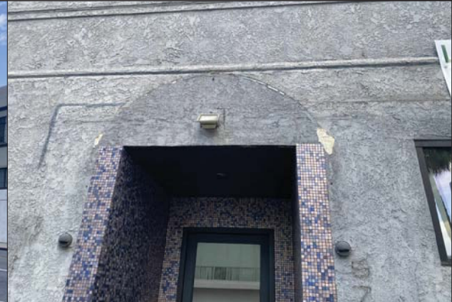
EXISTING ENTRY TO PROPERTY
