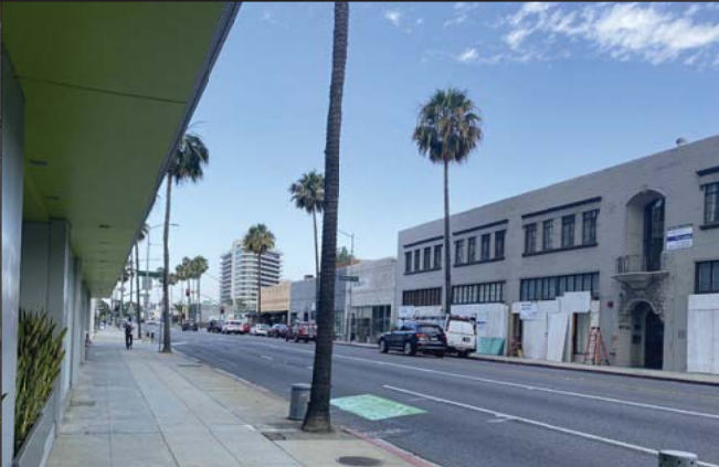
ADJACENT 9701 BLDG. UNDER REMODELING
